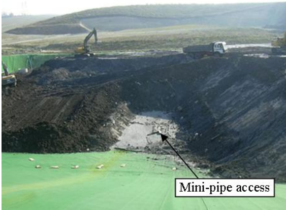
Figure 5. Filling with waste around the test pad
