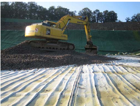
Figure 1. Putting into place of gravel on the geocomposite
