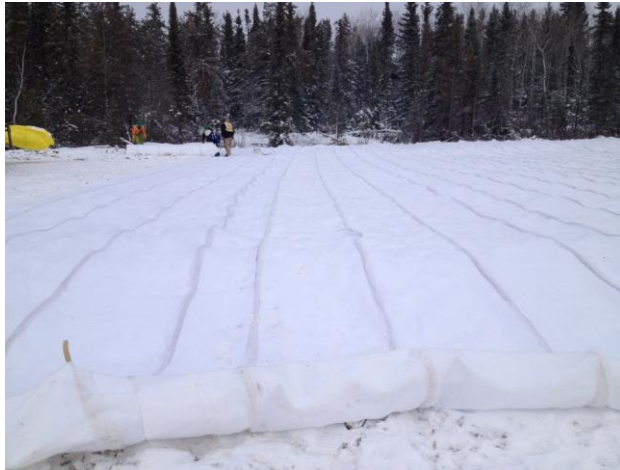
Figure 11. Drain tubes installation
