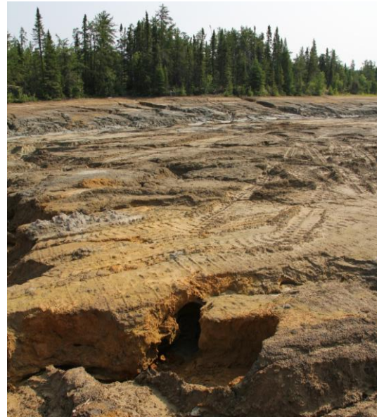
Figure 9. Silty clay backfill material
