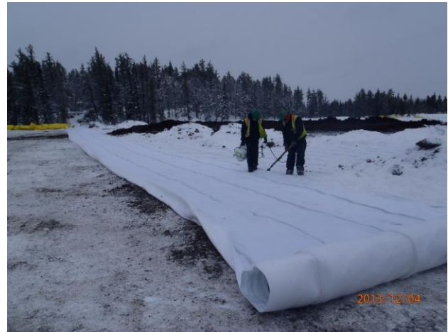
Figure 10. Unrolling drain tubes on frozen backfill
