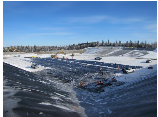
Figure 7. General view of tailing pond during construction
