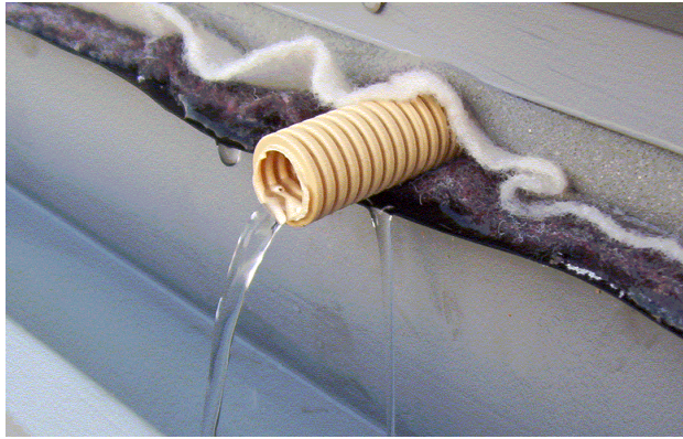
Figure 4. Drain tubes geocomposite water drainage
