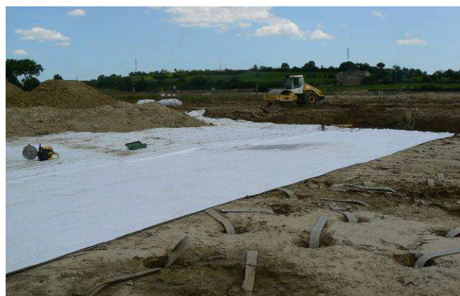
Fig. 4. Drainage geocomposite installation
