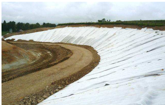
Fig. 6. Drainage mask construction with drainage geocomposite
