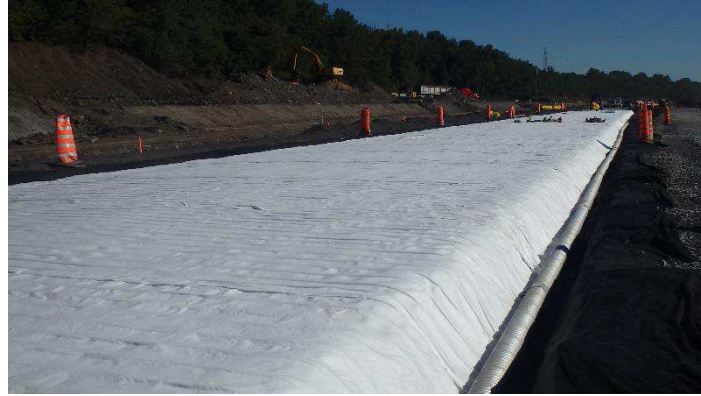
Fig. 11. Installation of the geocomposite
