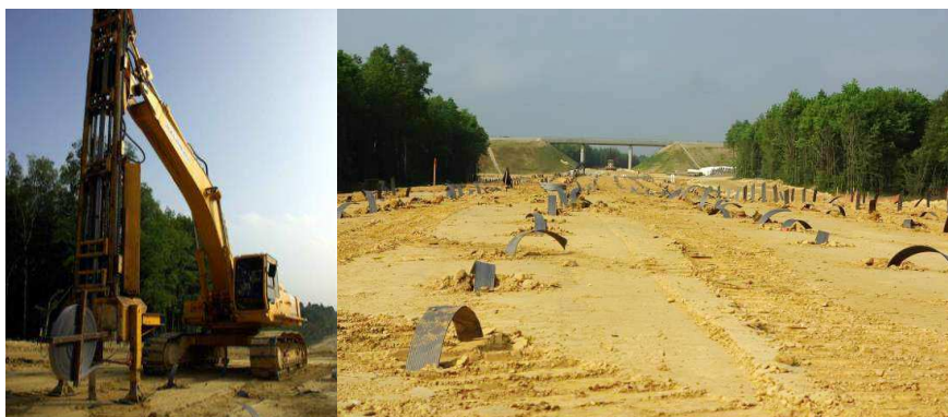
Fig. 3. Installation of the vertical wick drains
