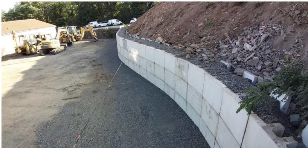
Figure 4. Test working site
