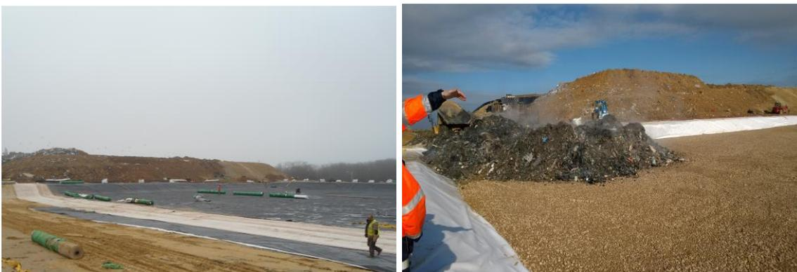
Figure 3. Installation of the geotextile reinforcement (Geoter® FPVA) and laying down of waste
