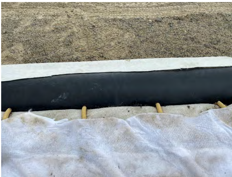
Figure 10. Mechanical connection of the geocomposite mini-pipes to the main header
