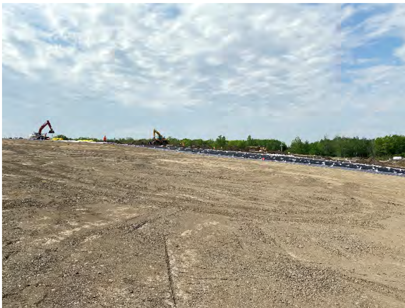
Figure 8. Soil surface conditions before the installation of the geosynthetics
