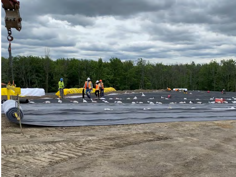
Figure 9. Installation of the multi-linear geocomposite for gas collection
