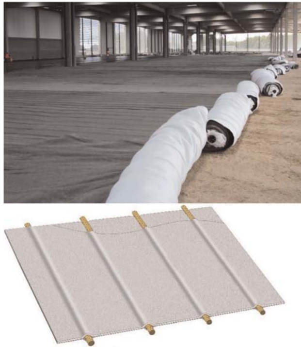
Figure 2. Installation of the geocomposite on the subgrade.
