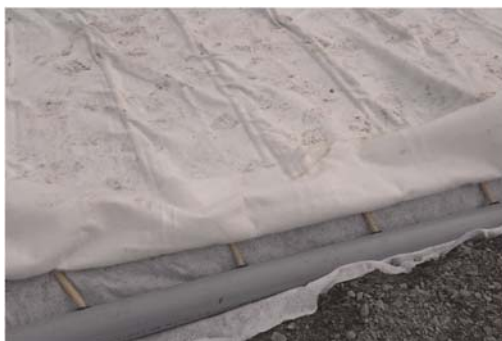
Figure 3. Connection to the header pipe.
