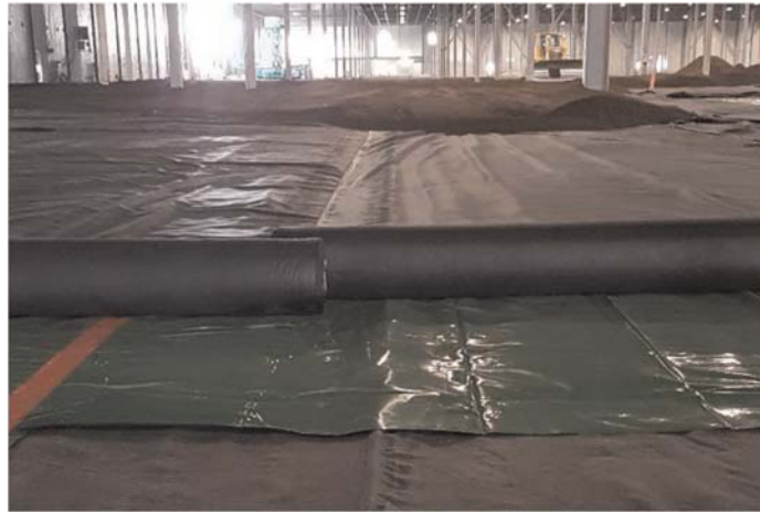
Figure 4. Vapor barrier and geotextile installation.
