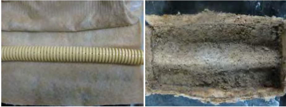
Figure 4 external and internal view of the geocomposite after 3 months of percolation of sulphuric acid
