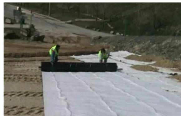
Figure 3. Installation of the geocomposite ant the top soil
