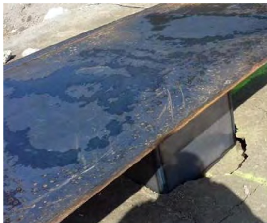
Figure 8. Steel plates on the steel cube
