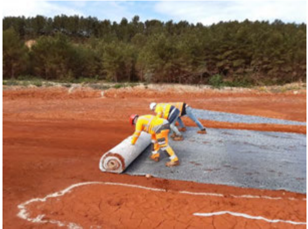
Figure 9. Continued installation of reinforcement geosynthetic
