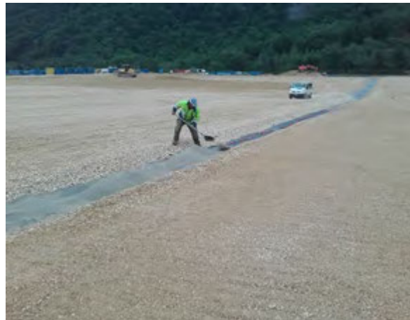
Figure 14. Backfilling of the gauges
