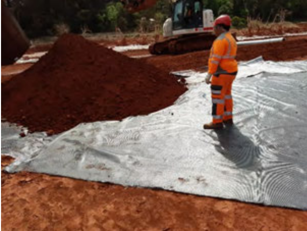
Figure 11. Placement of bottom ash soil over geosynthetic
