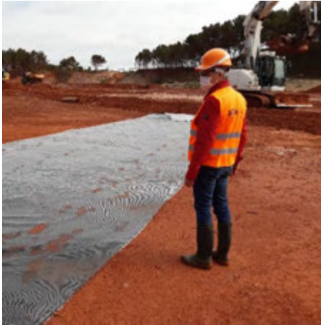
Figure 8. Installation of reinforcement geosynthetic
