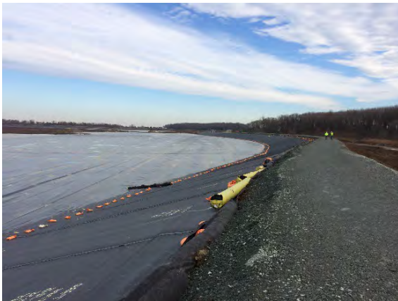
Figure 3. Site photo of deployed geotextile
