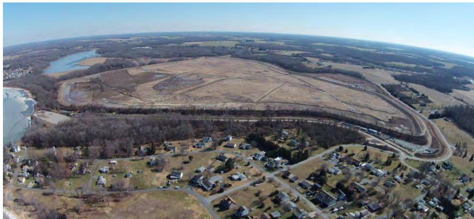
Figure 6. Aerial photograph of the Pearce Creek Disposal Facility
