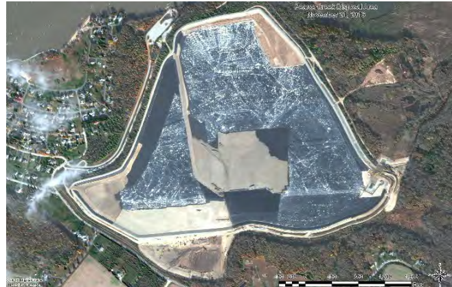
Figure 2. Aerial photograph of the site
