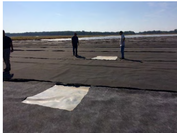
Figure 4. Photo of geotextile being sampled
