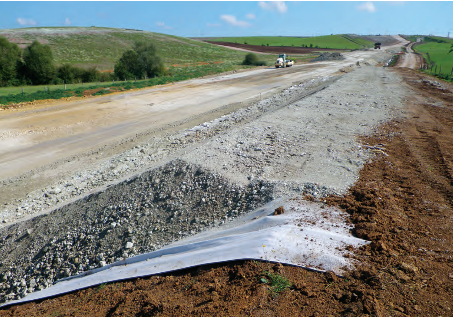
FIGURE 6 Drainage geocomposite installation on slope
