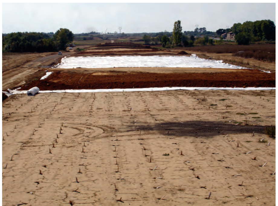
FIGURE 5 Installation of the vertical wick drains followed by DRAINTUBE
