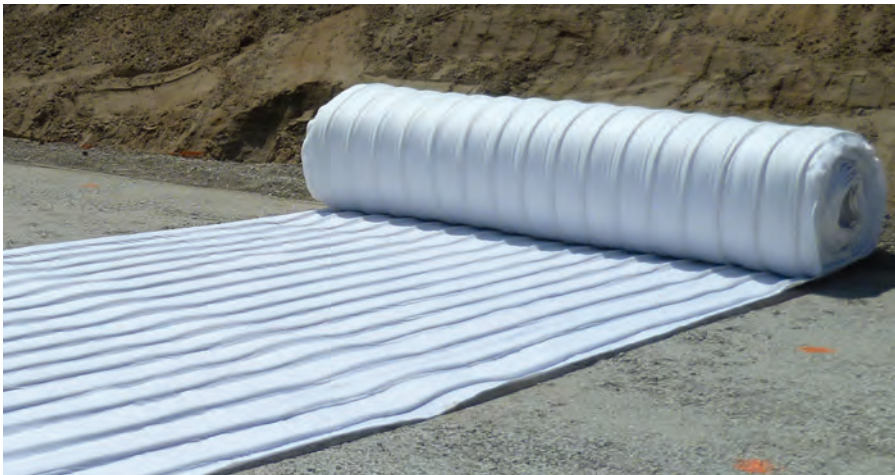
FIGURE 3 Unrolling of the DRAINTUBE geocomposite
