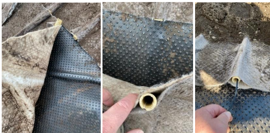
Fig. 11. Exposition of the geocomposite and the liner. Endoscopic inspection of the mini-pipes.
