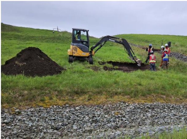
Fig. 9. Location of the exhumation and removal of the soil on top of the geocomposite.
