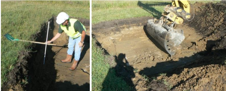
Fig. 3. Removal of the topsoil on top of the multi-linear drainage geocomposite.
