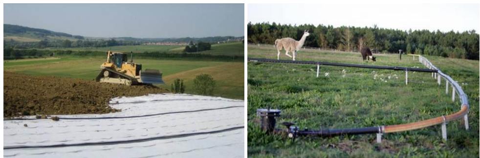
Fig. 1. Placement of topsoil over multi-linear geocomposite drainage and final vegetation cover.
