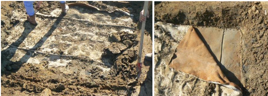
Fig. 4. Manual exposition of the two faces of the geocomposite.
