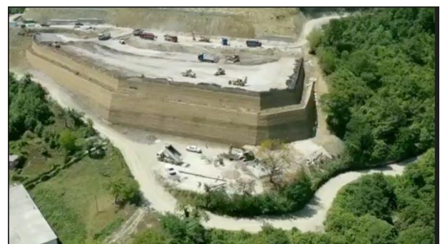
Aerial view of the retaining wall
